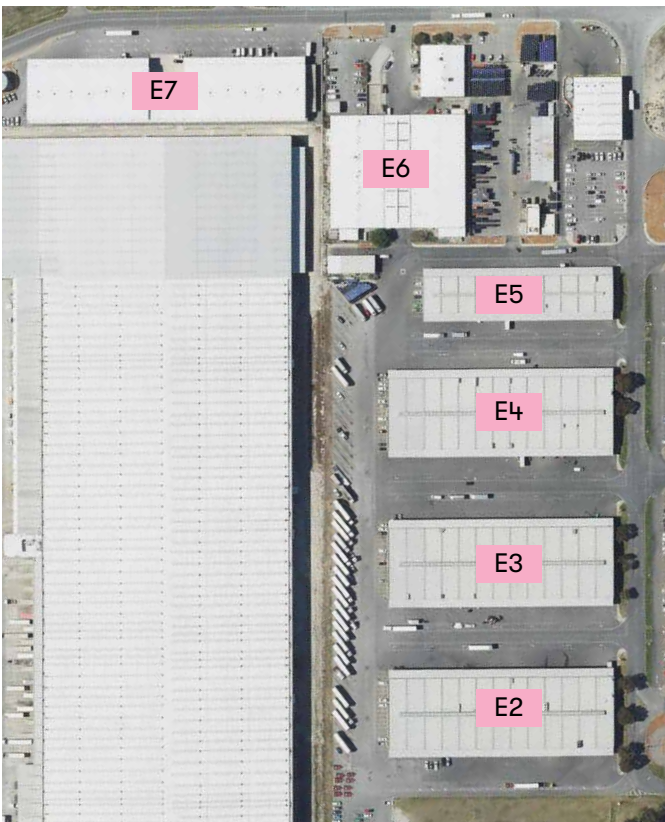
FIGURE 16 • Aerial view of warehouse precinct E
