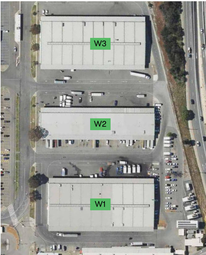
FIGURE 14 • Aerial view of warehouse precinct W
